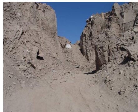
Figure 2. Main chineh entrance to Arge Bam located on the south side of the compound has been restored (left) with mud straw render restricting layered movement joints.
