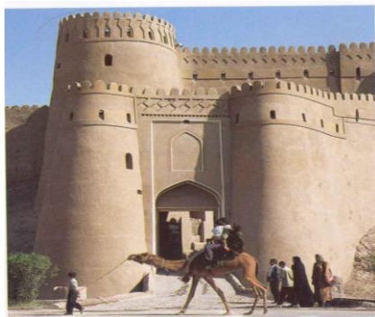
Figure 2. Main chineh entrance to Arge Bam located on the south side of the compound has been restored (left) with mud straw render restricting layered movement joints.
