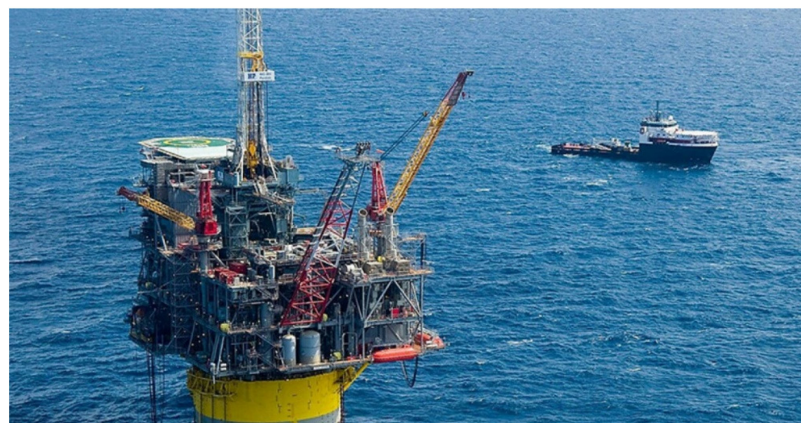
Figure 12. Perdido deep water SPAR platform in the Gulf of Mexico (GoM), (Courtesy: Statoil).
