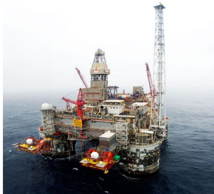
Figure 17. Heidrun Tension Leg Platform (TLP). (Courtesy: Statoil.).
