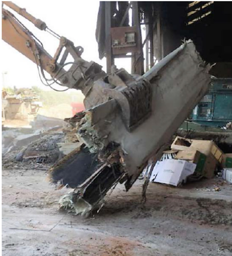
Fig. 22 Wind turbine blade waste disposal. Courtesy: Agecko.
