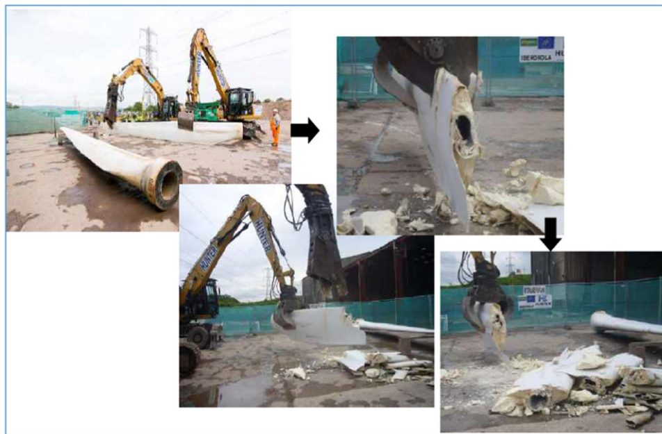
Fig. 17 Mechanical recycling of wind turbine blades after demolition, in pretreatment stage. Courtesy: Source: Estevez, D.G., 2019. Demonstration of wind turbine rotor blade recycling into the coal clough windfarm decommissioning opportunity. In: Proceedings of the Wind Europe Conference & Exhibition, 2-4 April 2019, pp. 1–16, Workshop On Blade Disposal. Bilbao: LIFE + Brio.
