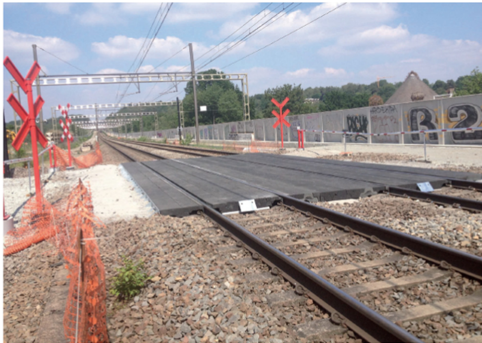
Fig. 25 Level crossing panels including recycled Glass Reinforced Polymer and phenolics from car parts. Courtesy: Reprocover.
