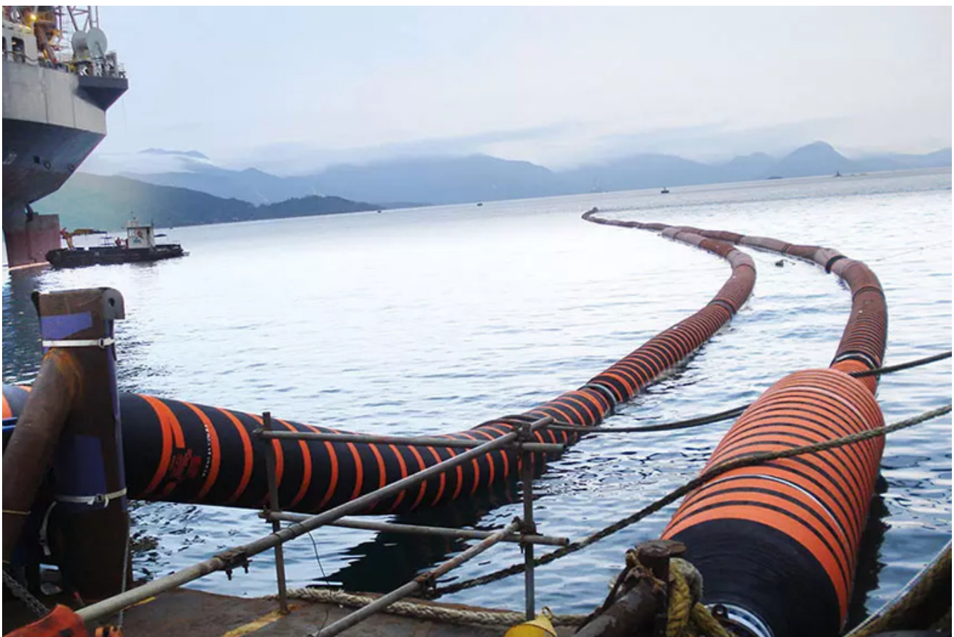
Figure 1. Trelleborg’s Sealine floating hose during installation to a supply vessel. (Sealine is a product type that is specifically designed for floating hose configurations, while Reeline is a product type that is specifically designed for reeling hose configurations. Both Sealine and Reeline are hose products made by Trelleborg, a hose manufacturer. Courtesy: Trelleborg; adapted with permission.).
