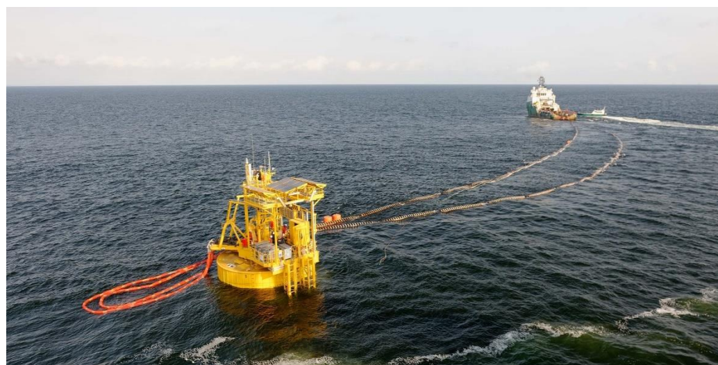
Figure 2. Full replacement operation of floating hoses, submarine hoses, hawsers and a single point mooring (SPM) buoy attached to a service offshore vessel (SOV) by a tug supply boat, located at 35 m water depth in Republic of Congo, Djeno Terminal (Courtesy: Bluewater & South Offshore [158]).
