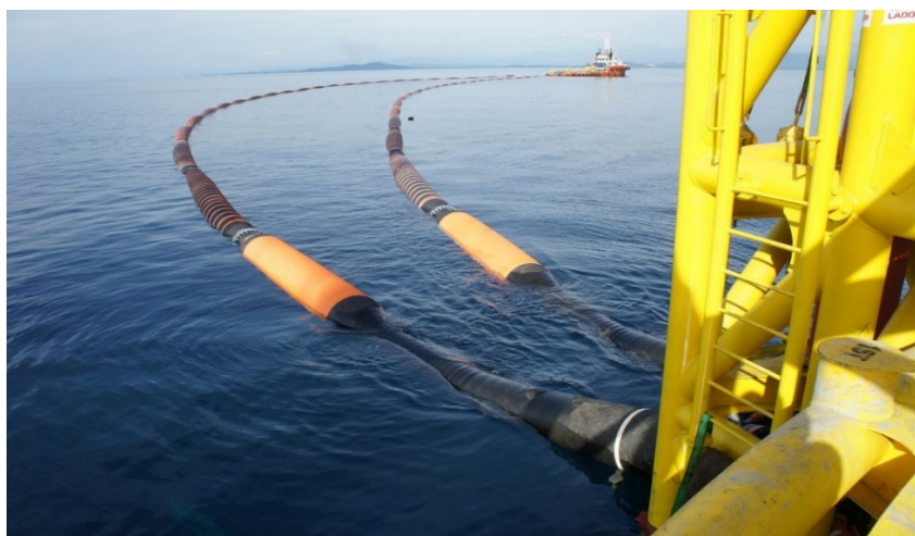
Figure 2. SPM buoy hose system from the buoy to the shuttle tanker on an SPM Terminal (Provided by Trelleborg for this paper, and used with permission, Courtesy: Trelleborg).
